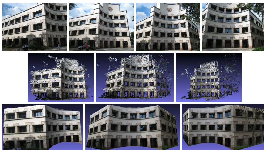
Fig. 5 Reconstructed mesh models of building 1. (Row 1) Sample images from various views. (Row 2) Point cloud recovered by PMVS and (Row 3) reconstructed textured mesh model at various viewing angles.
